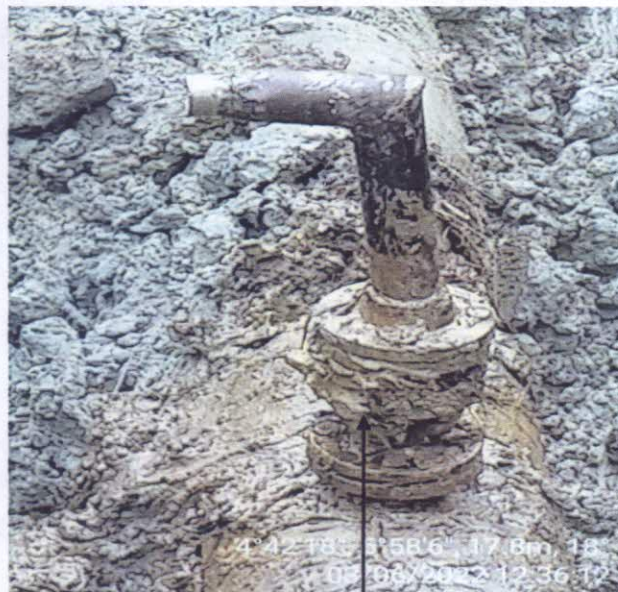
SPILL POINT (After excavation: Installed 3" ball valve At 12 O'clock position on the pipeline)
